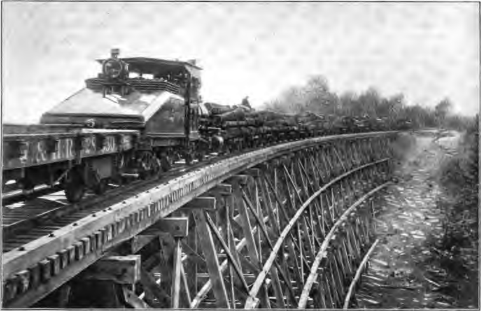
AN ALGOMA CENTRAL LOG TRAIN ON THE ROOT RIVER BRIDGE.
